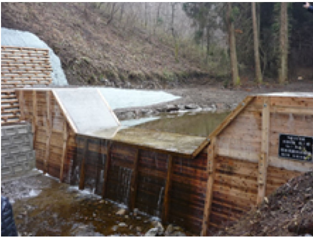
Fig. 4 Concrete check dam with timber forms left in place
